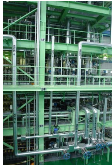
Fig. 1. Schematic diagram of the average BDFT installation in the primary pipes of the ATLAS.
